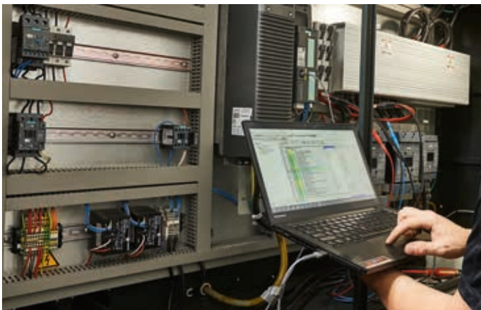
Thanks to the integrated web server, it is possible to display operating data, maintenance and fault messages on a PC.
