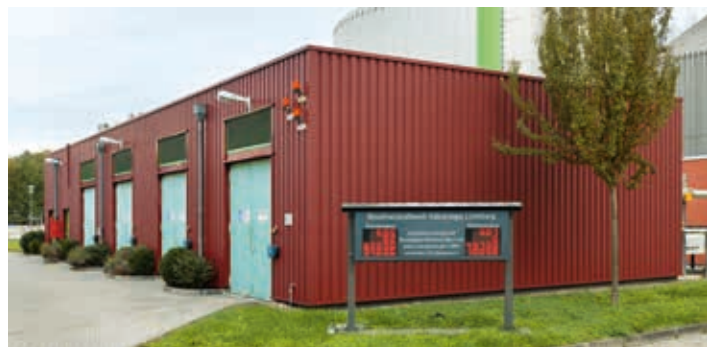
The illuminated panel shows the current values of the energy produced from the wastewater sludge.
