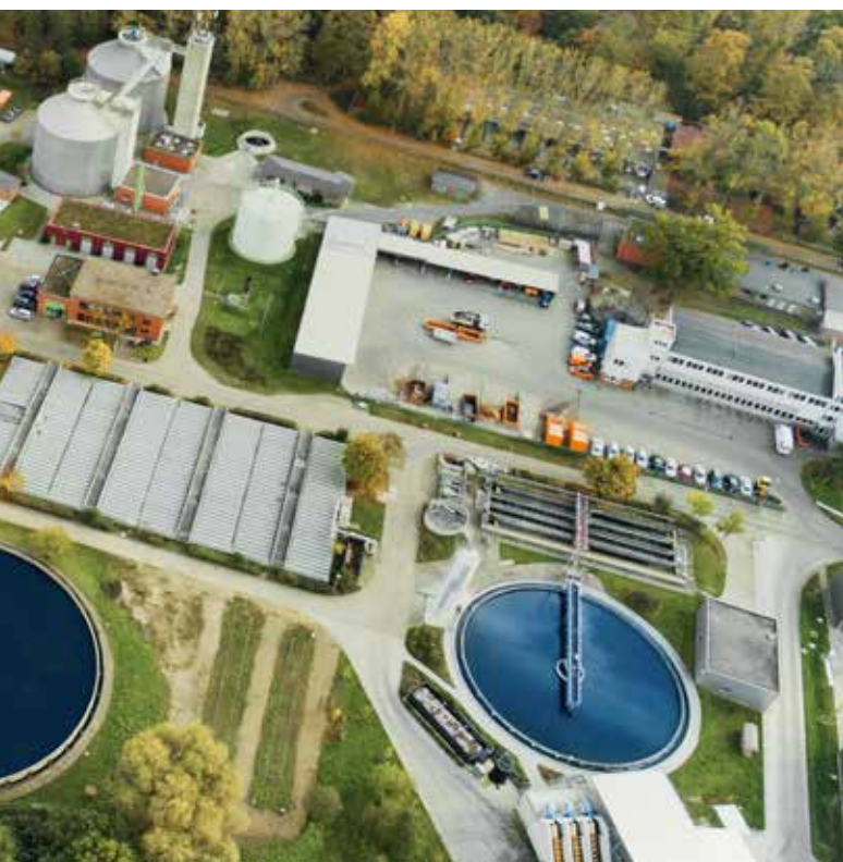
A bird's eye view of the Lüneburg wastewater treatment plant.
